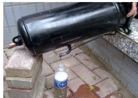
Figure 6-2.8: Draining oil from a compressor
