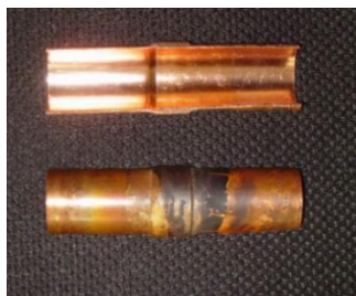
Charge N2 to the pipes
